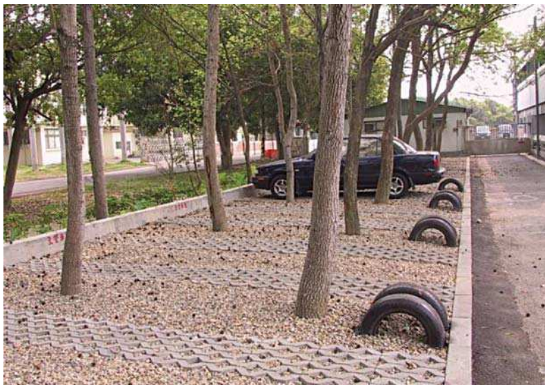
7.9. An example of permeable pavement improvement project in Green Remodelling Project, 2003. (Source: Author)
