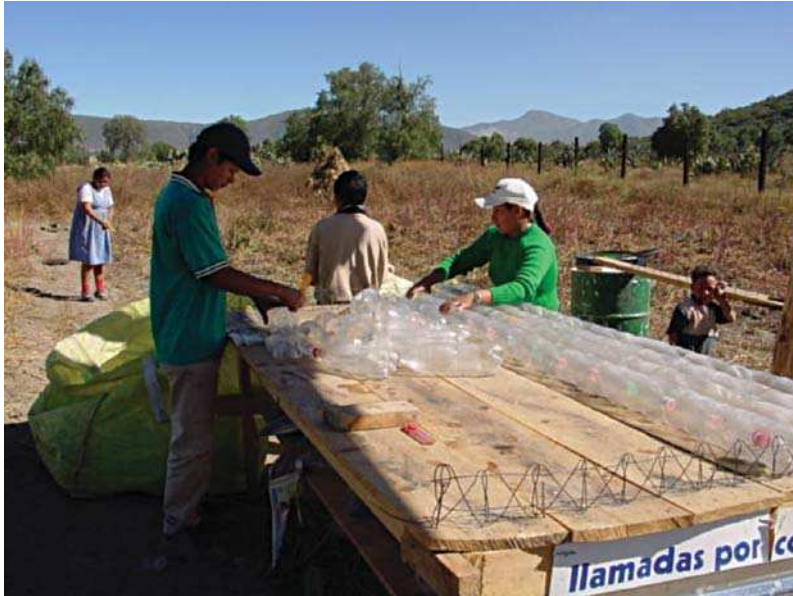
13.8. PET panels construction process. (Source: Author)
