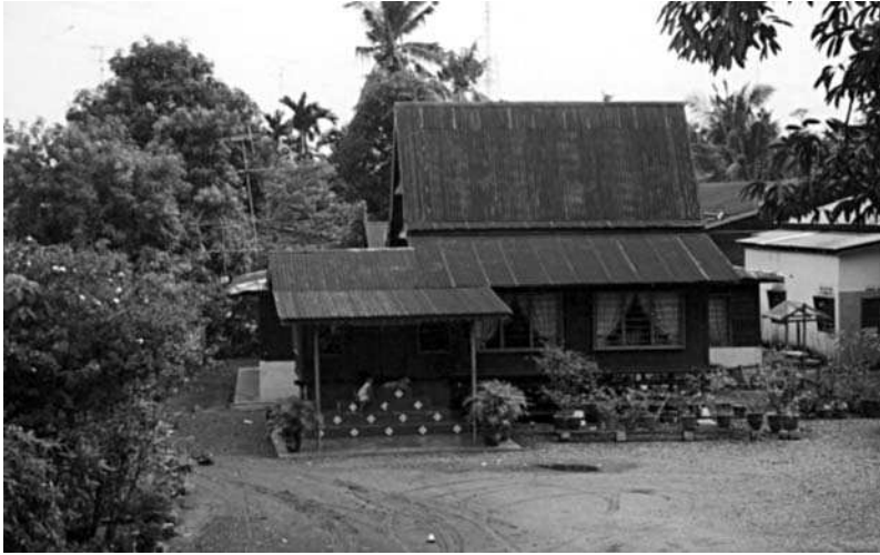
14.5. Kampong House, Malaysia. (Source: Author)
